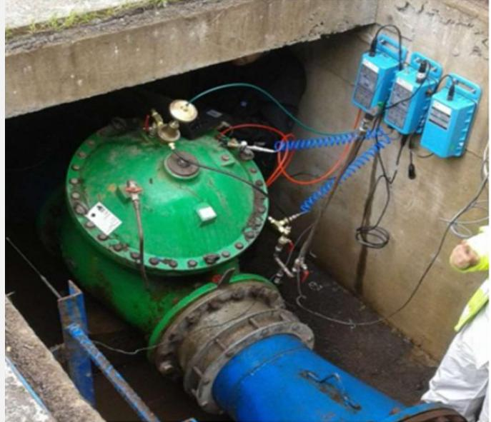
Fig 1 – PRV Controller Installed
